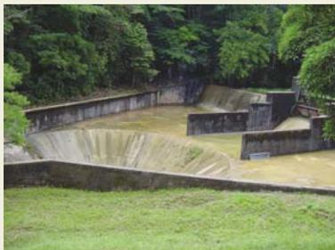
The reservoir was constructed by damming the Quare River, which enters the reservoir in a majestic split series of waterfalls that constantly replenish the lake from which an unfailling supply is drawn.
