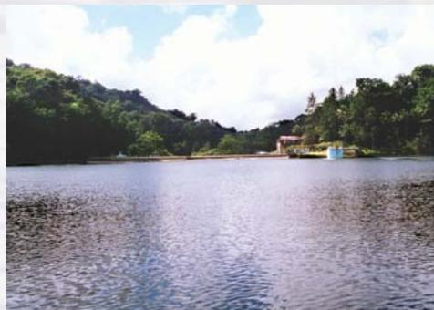
The reservoir reaches its maximum depth at 20 metres (65 feet) and has an approximate capacity of 4,750,000 cubic metres or just over one (1) billion gallons. It is also capable of producing 38,180 cubic metres of water per day (8.4 m.g.d.).
