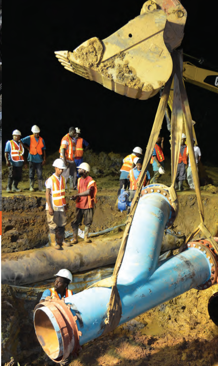
Navet Trunk Main Project
