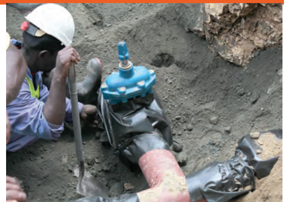
Sluce valve installation at the Courland to Buccoo Pipeline Project
