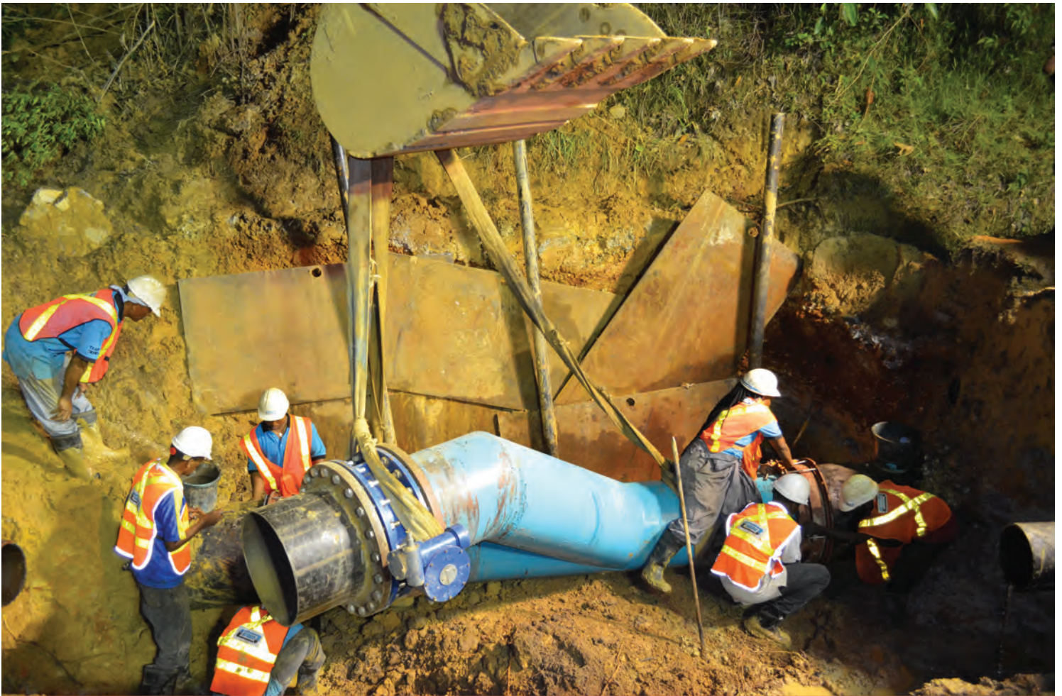
Workers position new transmission line at Quare, Valencia
