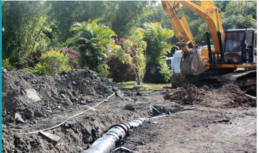
A 16 inch ductile iron pipe being installed at Courland Water Treatment Plant (Courland to Buccoo Pipeline Project)
