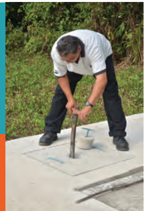
Systems Operator, Mitra Ragoonan demonstrates how the valve is accessed at the Sangre Grande Pressure Reducing Valve Chamber.
