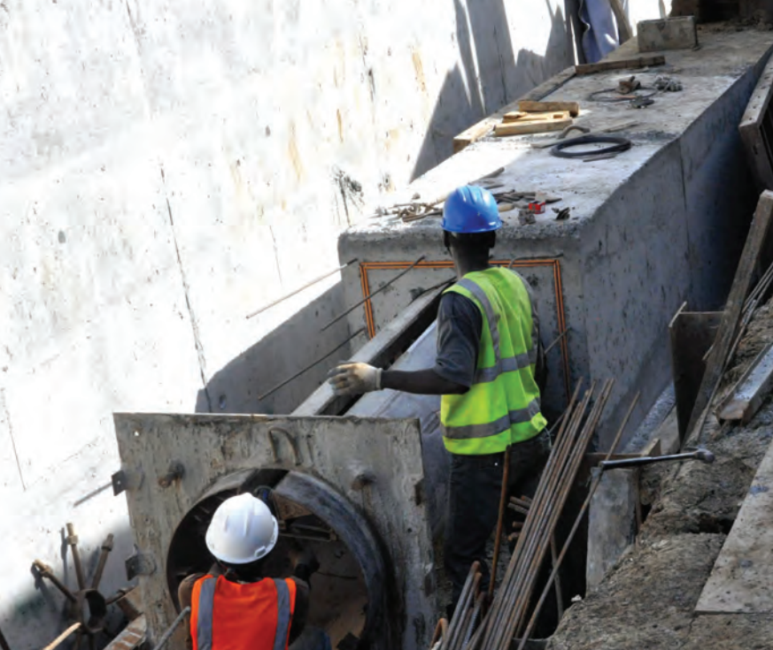
Thrust blocks being constructed at the Vistabella Sewer Main Replacement Project
