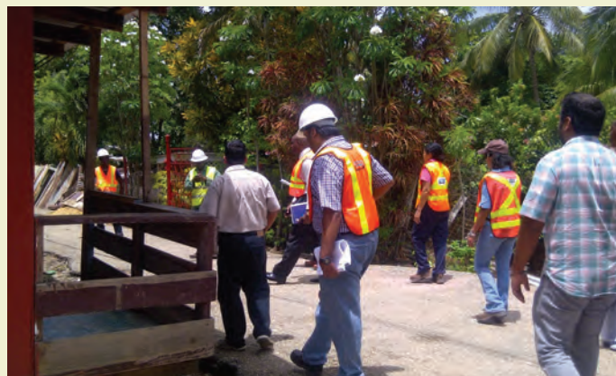
Wastewater Project Team walking the trunk routes in San Fernando with Surveyors to confirm location of manholes. (IDB loan, No. 2890/OC-TT)
